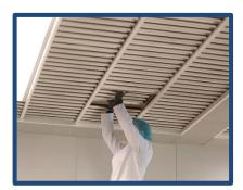
7 – Place the cassettes back into the grid and push together until the row is full (max. 10 cassettes).
