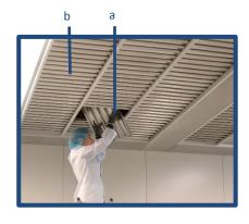
2 – Lift the cassettes carefully out of the C-profiles. Handle the cassettes on the side (a) or on the small register (b) only.
